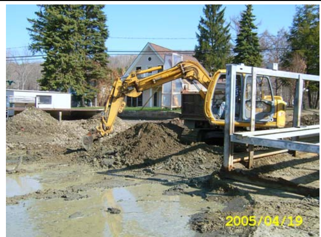
Sediment removal – also done in 2006
